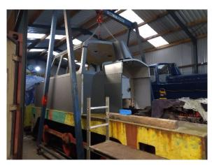
With this task completed the single piece cab top half was craned into place, each bolthole individually lined up and bolts fitted, and when all was satisfactory it was bolted down tight.
